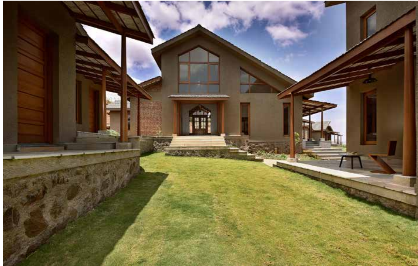
↑ View of the Kid's Block and Master Block on either side with the Living Block.
